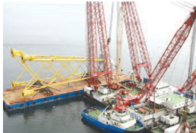
First jacket being prepared for installation
