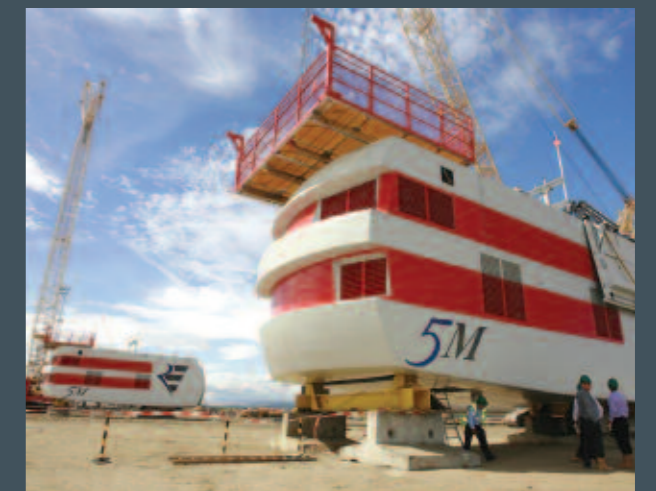
The two wind turbines in the Nigg construction yard
