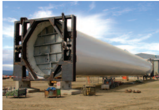
Tower being assembled at Nigg fabrication yard.
