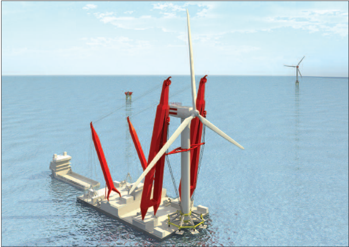
Figure 7.2 Assembled turbines and towers arriving at offshore location.
