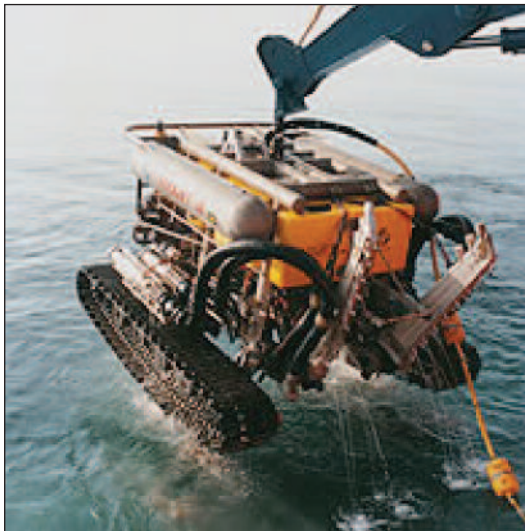
Figure 8.1 Example of the type and size of machine that would be used to fluidise the seabed for the burial of the umbilicals.
